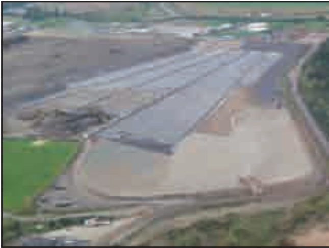
Figure 6.1 Installation of liner at MSW landfill
