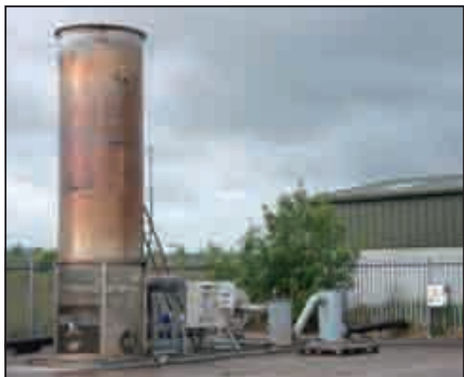
Figure 8.1 Enclosed flare
