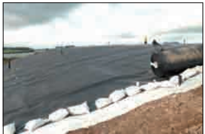
Figure 7.2 Installation of final cap at MSW landfill
