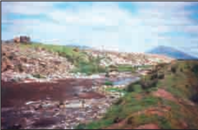
Figure 2.5 Poor environmental management at MSW landfill in 1997
