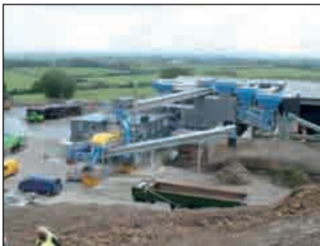
Figure 4.2 Overview of Waste Transfer Station
