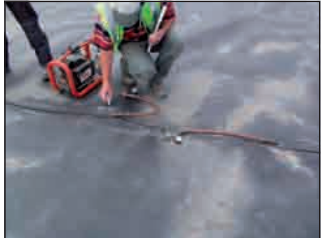
Figure 6.2 Testing of welds on liner at MSW landfill
