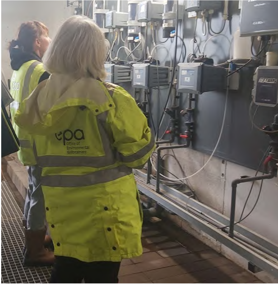
Figure 3.2: Water treatment plan inspection
