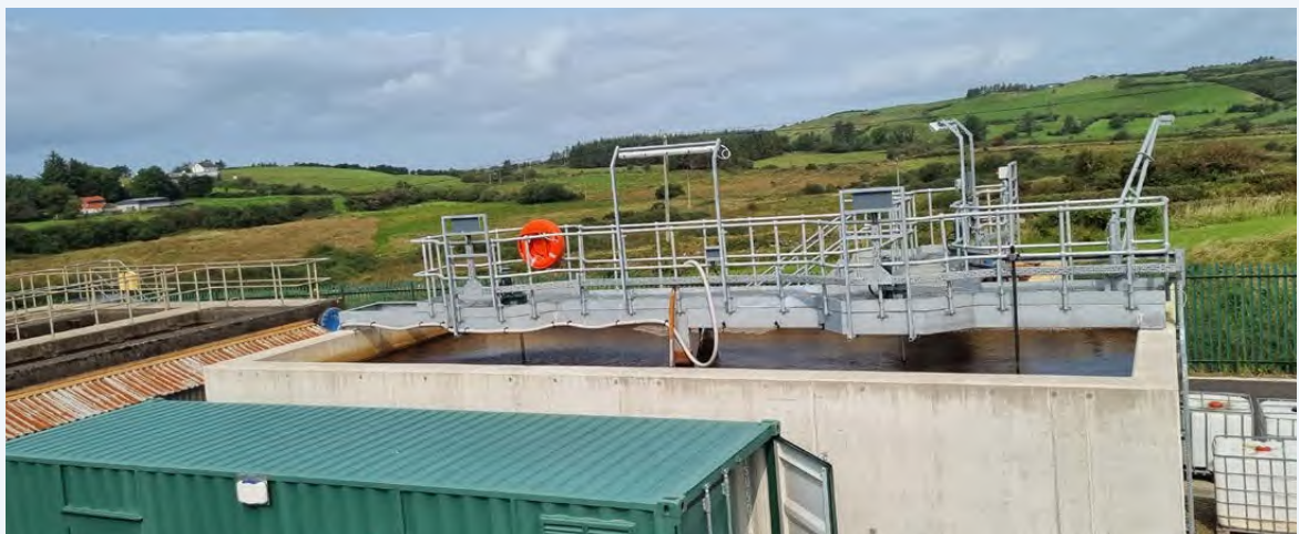
Part of West Clare Water Treatment plant
