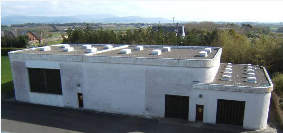
Cavanhill WTP (Chemicals building)
