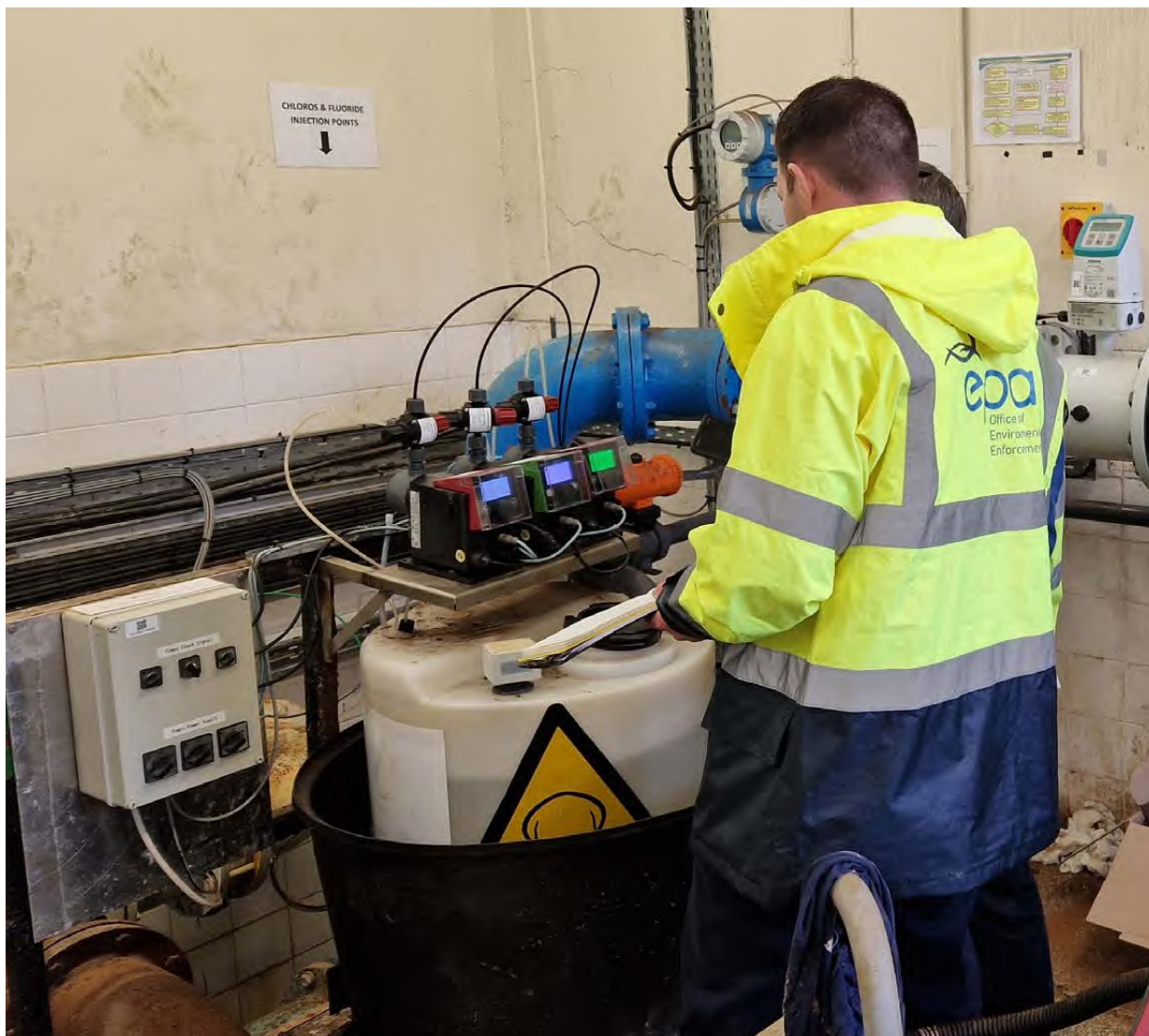
Figure 4.4: Inspection of water treatment plant dosing equipment
