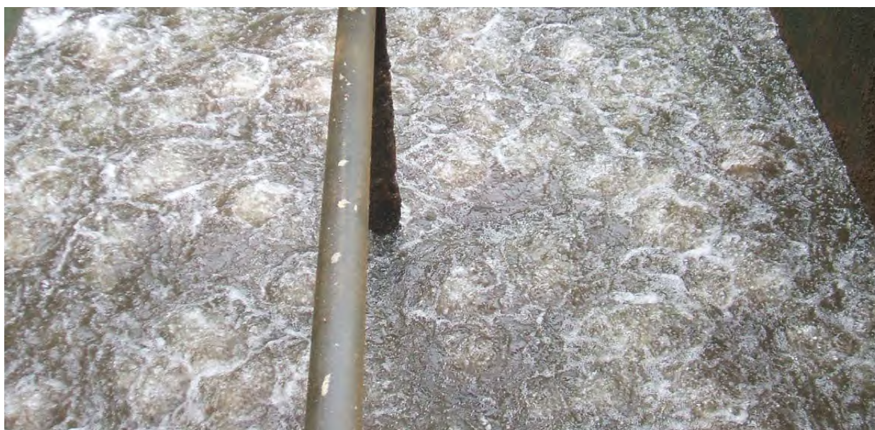
Figure 3.4: Inspecting a water filter (uneven distribution of bubbles means there is a problem with this filter).
