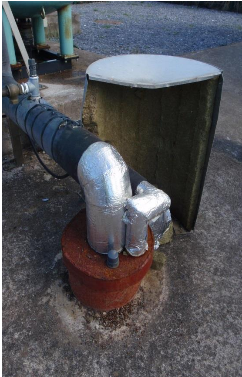
Figure 5: Wellhead constructed above ground level and borehole fully capped and sealed
