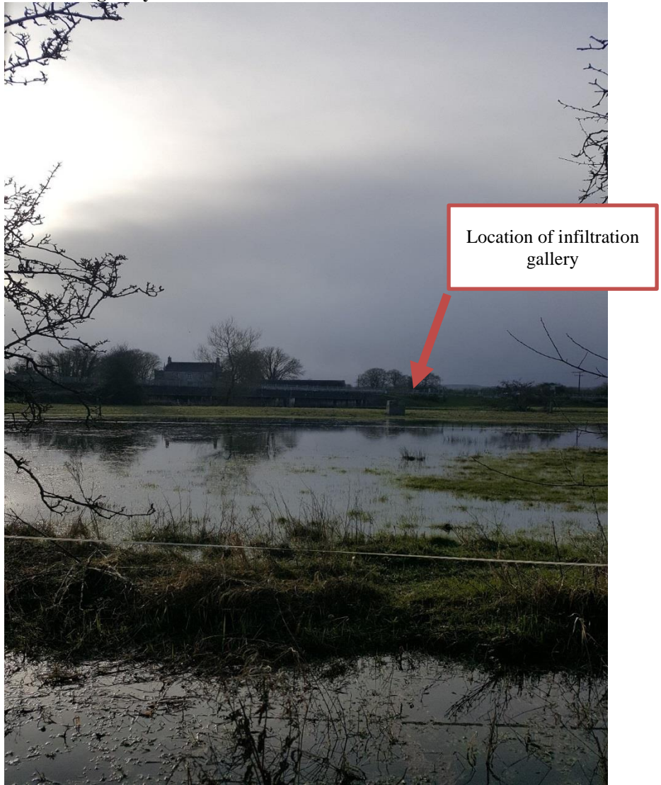
Photo 1: View of infiltration gallery from the water treatment plant. Land is flooded around infiltration gallery.
