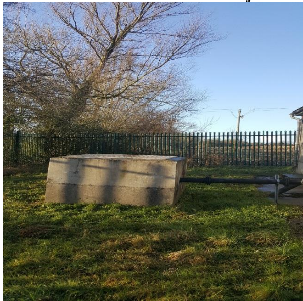
Photo 2: Raw water collection chamber adjacent to water treatment plant.
