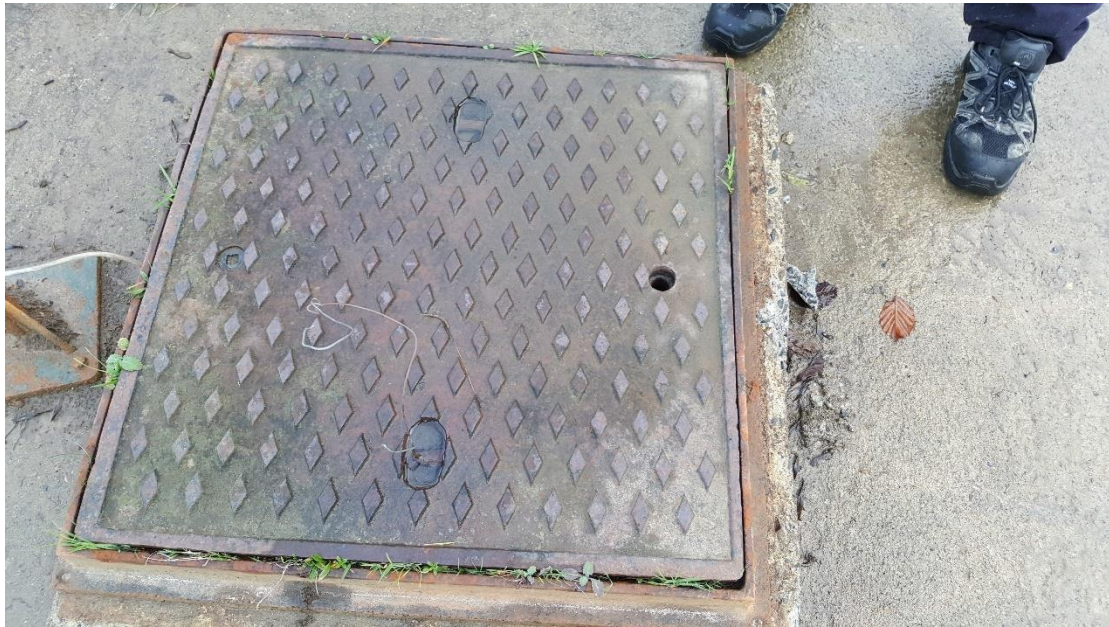
Photo 3 Inspection hatch on Cherrymount Reservoir
