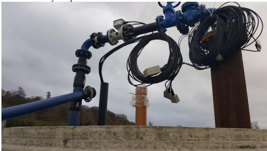
Photo 2: Partially completed Borehole No. 4 well head.
