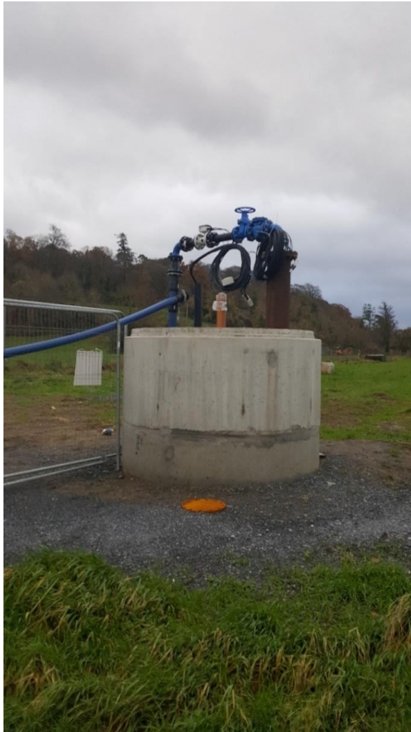
Photo 2: Partially completed Borehole No. 4 well head.
