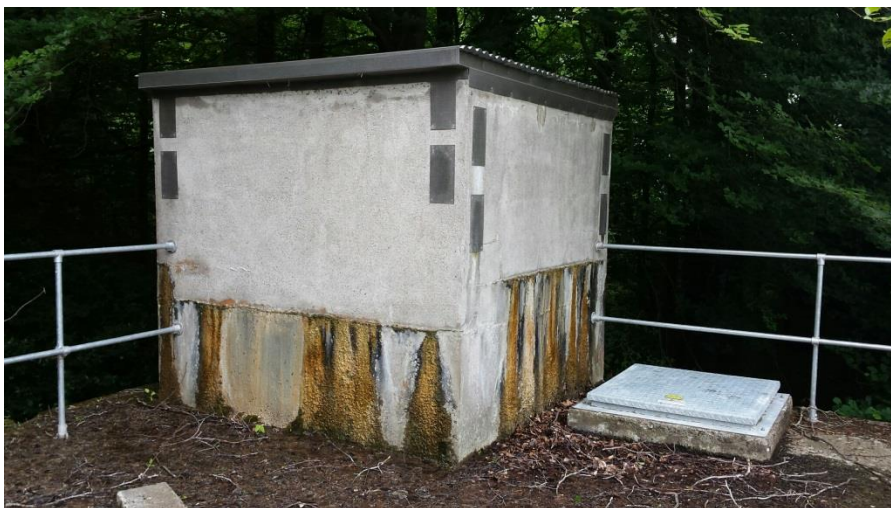
Photo 3: Recent upgrade works to the reservoir's plate aerator housing structure
