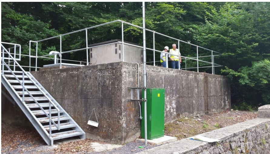
Photo 2: Cork Road Reservoir
