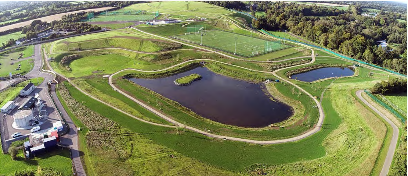
Remediated landfill Kerdiffstown
