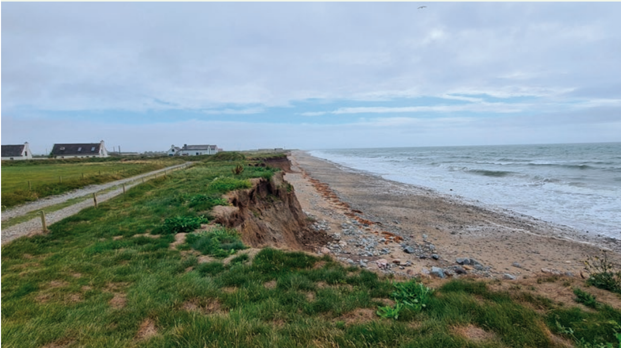
Figure 5.12 Coastal erosion near Kilmore, Co. Wexford
