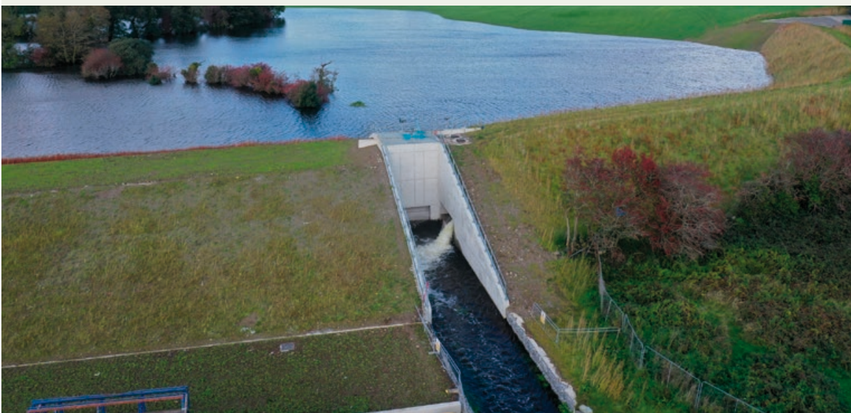
Figure 4.13 Clonakilty flood relief scheme – retention infrastructure
