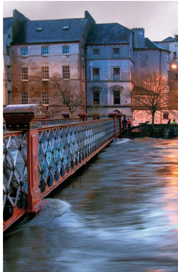
High water levels at St Vincent's Bridge, Cork City
