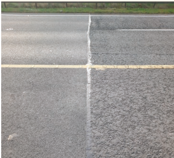
Figure 3.6 Lower noise road surface using stone mastic asphalt (left) and traditional coarse road surface using hot-rolled asphalt (right) on the M4 near Kilcock, Co. Kildare.
