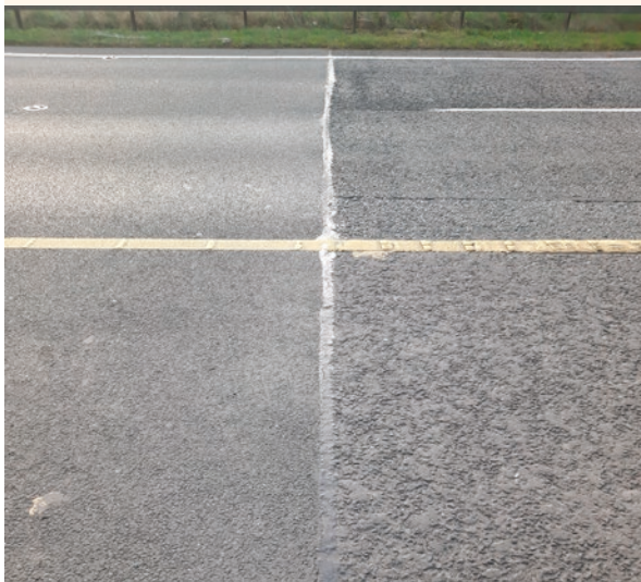
Figure 3.6 Lower noise road surface using stone mastic asphalt (left) and traditional coarse road surface using hot-rolled asphalt (right) on the M4 near Kilcock, Co. Kildare.
