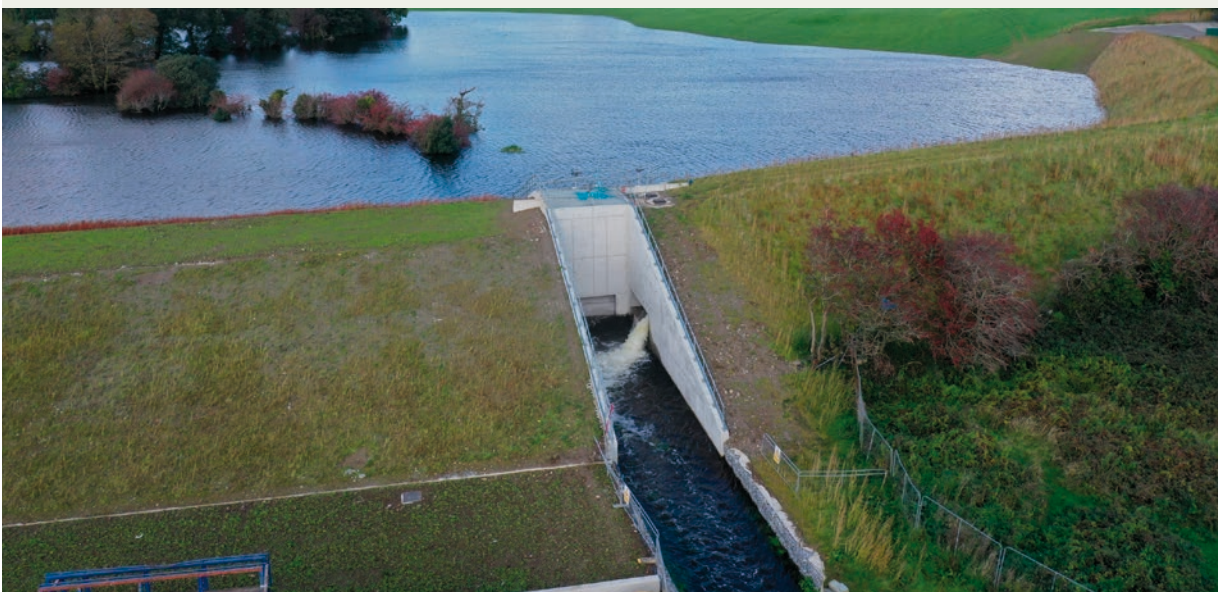
Figure 4.13 Clonakilty flood relief scheme – retention infrastructure
