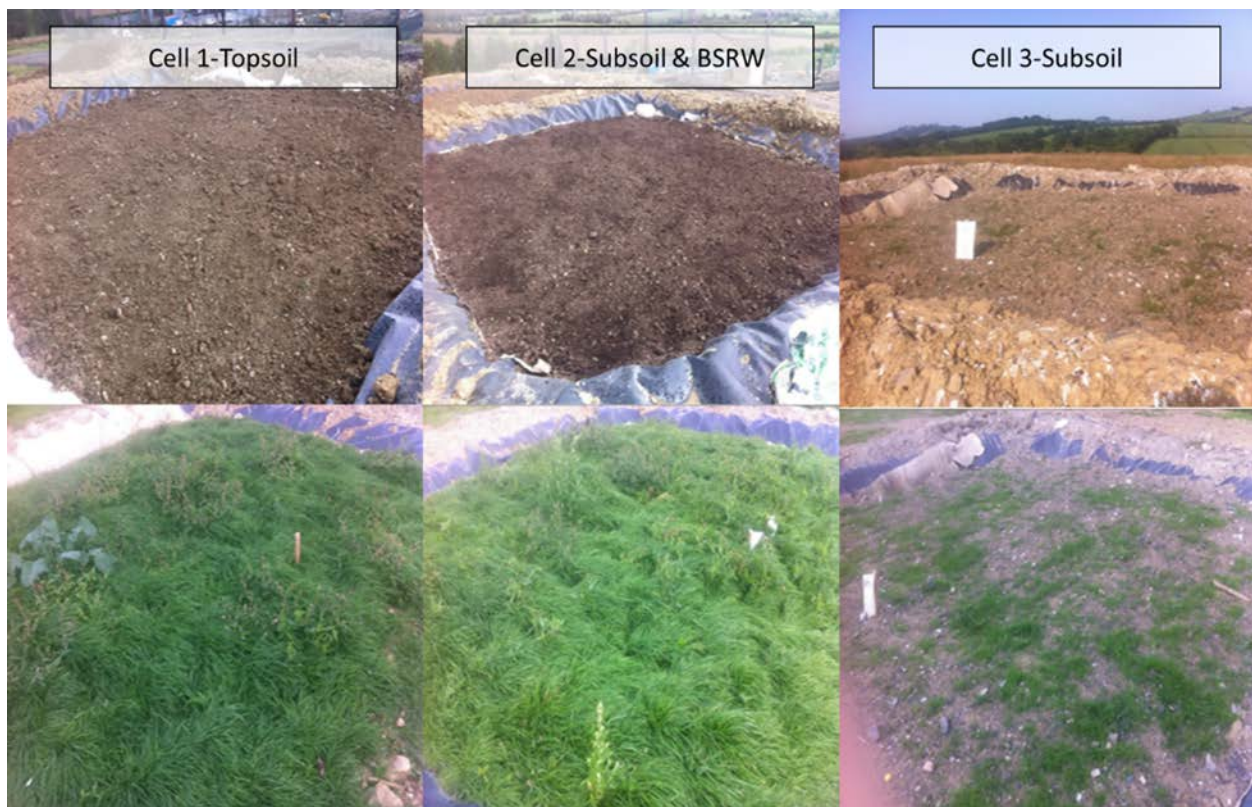
Figure 8.1. View of the three landfill capping cells at installation and establishment of grass in 2013.
